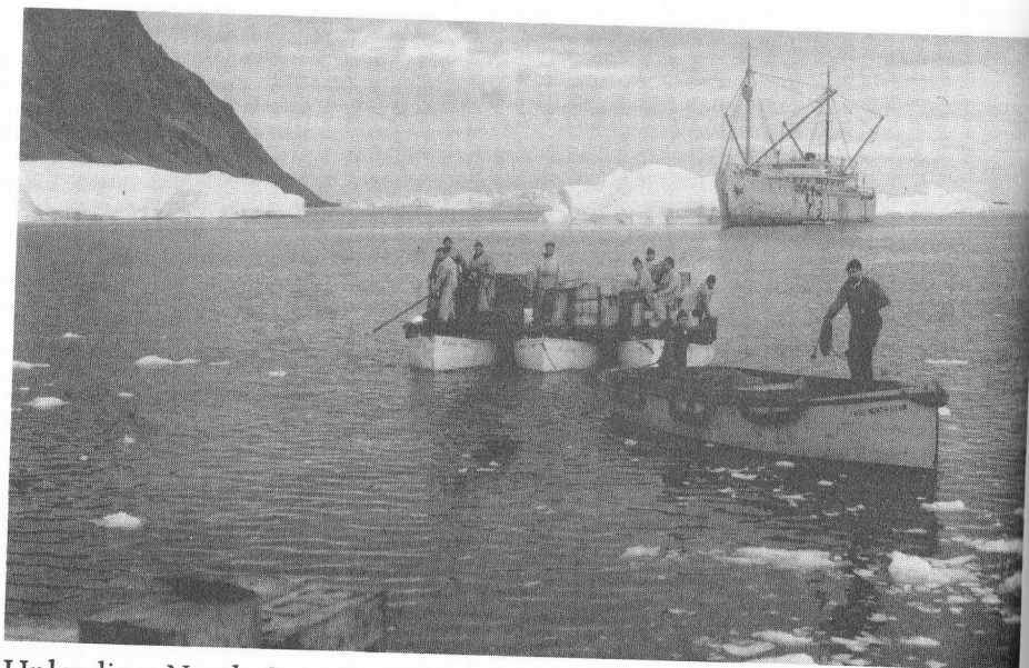
Unloading North Star , East Base from ship to Stonington Island on a barge.
