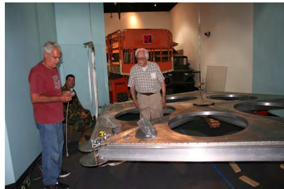
Lee Mattis, left, and John Perry, far right, assemble the hardware used to hang the top section of the South Pole Station Dome from the roof of the new Seabee Museum in Port Hueneme, California. Mattis, Perry and Jerry Marty worked for years to save the Dome and see it enshrined in a museum.
