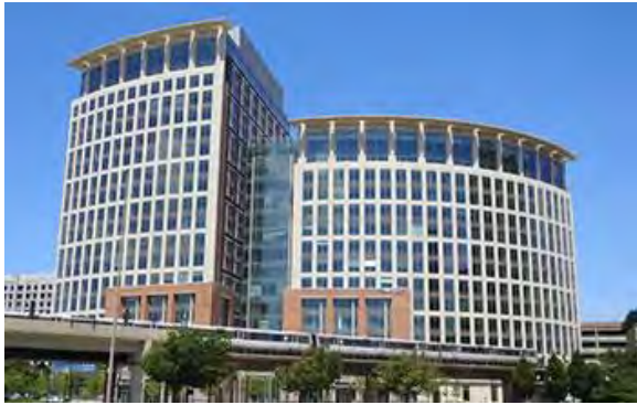
The new National Science Foundation building in Alexandria, Virginia
