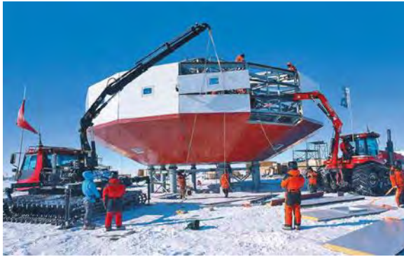
Taishan Station, East Antarctica, under construction
