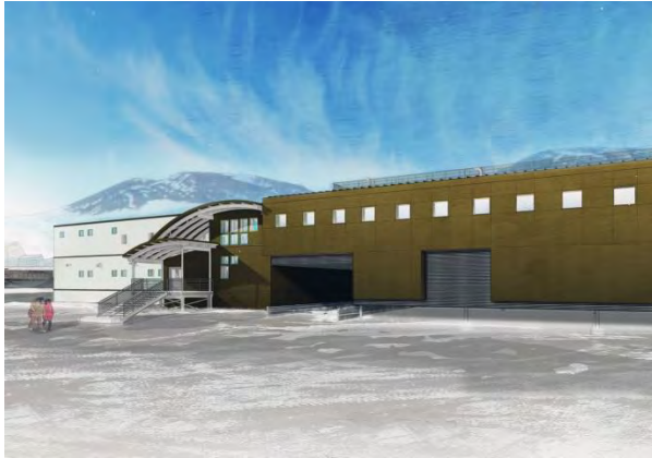
Information Technology and Communications building going up at McMurdo. Photo by Ferraro Choi.
