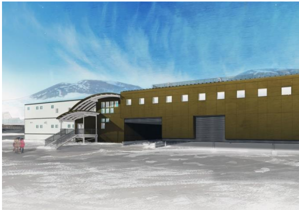
Information Technology and Communications building going up at McMurdo. Photo by Ferraro Choi.
