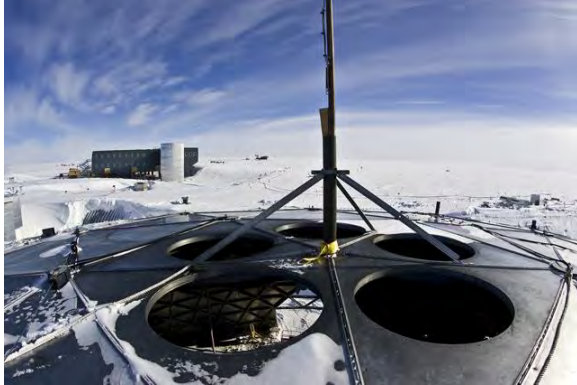
In Antarctica at the South Pole, the top of the Dome is shown in its environment, while the dome station was still in operation. Station buildings were under the dome. The new (dedicated 2008) elevated station is in the background.
