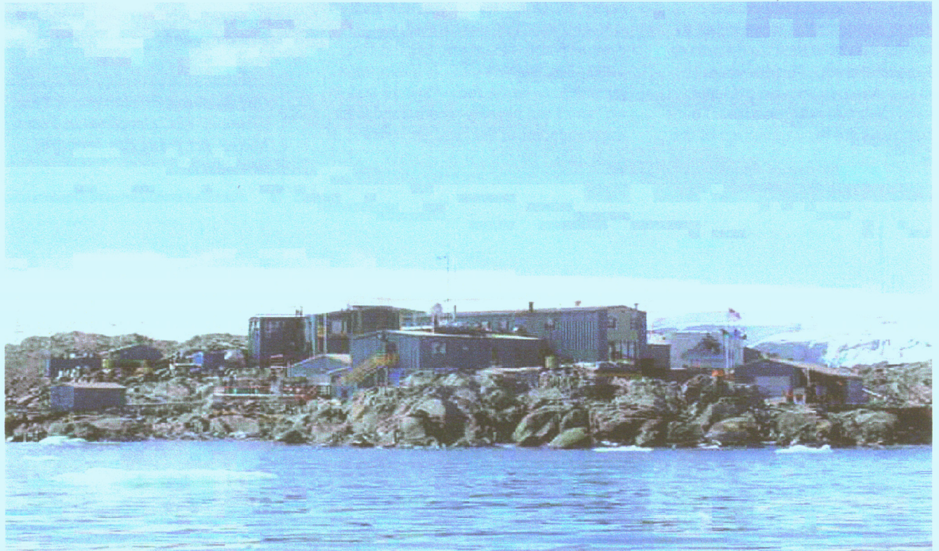
Figure 3: Palmer Station (above)
